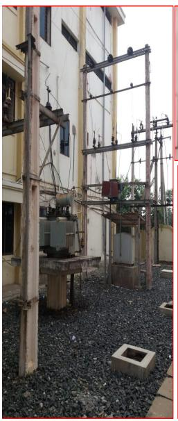
250 KVA, 415 V, 11 KV **TRANSFORMER** CONTRACTED MD: 225 KVA SOLAR POWER CAPACITY: 160 KW
